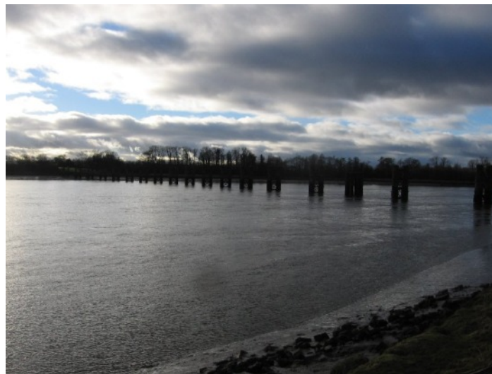
The old railway bridge
